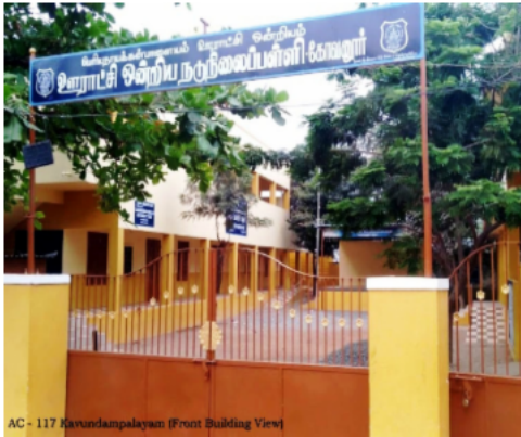
AC - 117 Karundampalayam (Front Building View)
