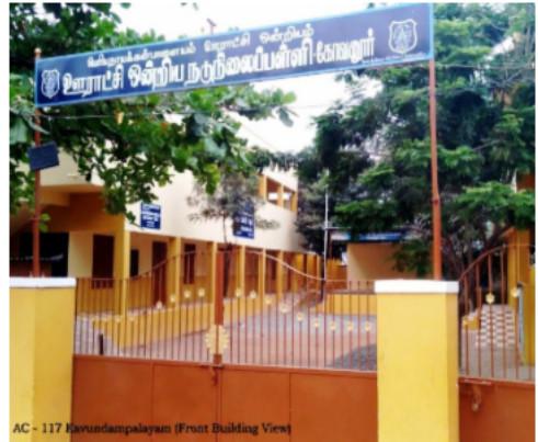
AC - 117 Karundampalayam (Front Building View)
