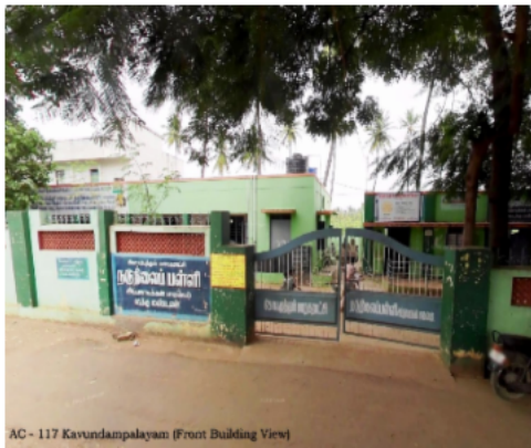
AC - 117 Kavundampalayam (Front Building View)
