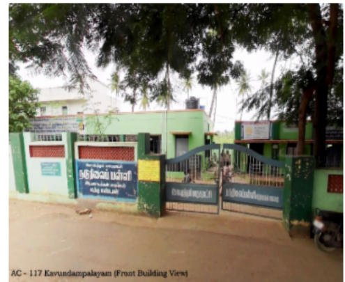
AC - 117 Kavundampalayam (Front Building View)
