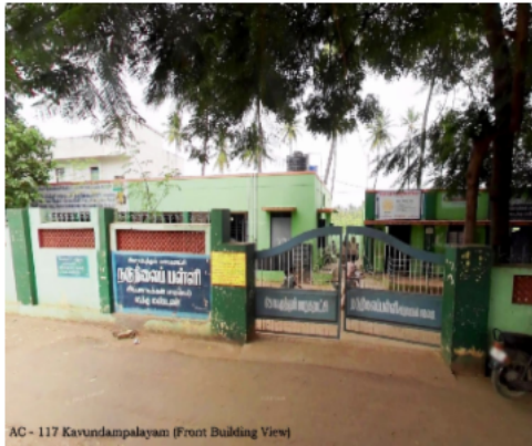
AC - 117 Kavundampalayam (Front Building View)
