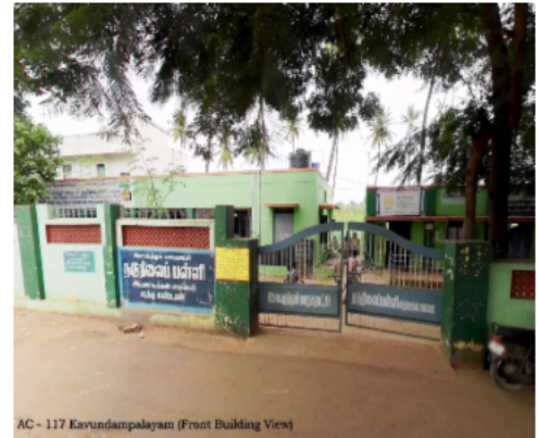
AC - 117 Kavundampalayam (Front Building View)
