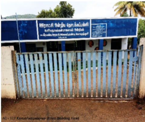
AC - 117 Kotturampalayam (Front Building View)
