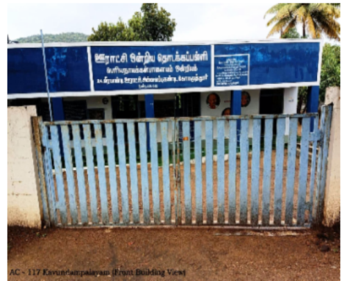
AC - 117 Kotturampalayam (Front Building View)
