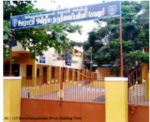
AC - 117 Kuvundampalayam (Front Building View)
