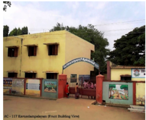
AC - 117 Kavundampalayam (Front Building View)
