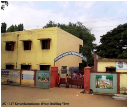
AC - 117 Kavundampalayam (Front Building View)
