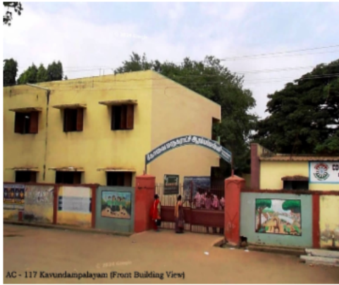
AC - 117 Kavundampalayam (Front Building View)
