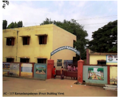
AC - 117 Kavundampalayam (Front Building View)
