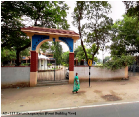
AC - 117 Kavundampalayam (Front Building View)
