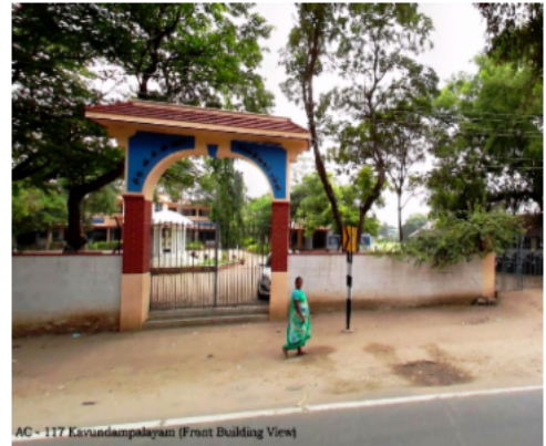
AC - 117 Kavundampalayam (Front Building View)
