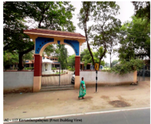
AC - 117 Kavundampalayam (Front Building View)
