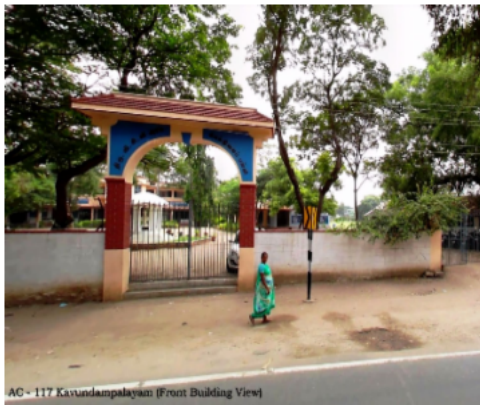
AC - 117 Kavundampalayam (Front Building View)
