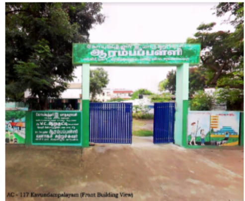
AG - 117 Kavundampalayam (Front Building View)
