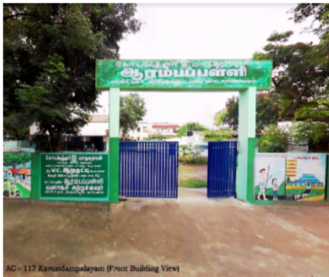
AG - 117 Kavundampalayam (Front Building View)
