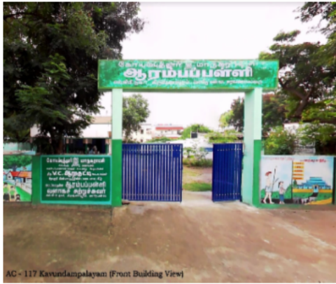
AG - 117 Kavundampalayam (Front Building View)
