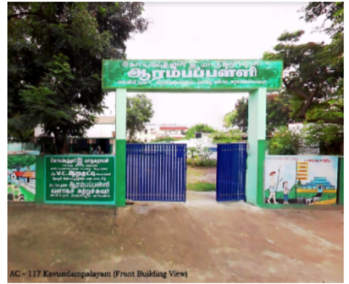
AG - 117 Kavundampalayam (Front Building View)
