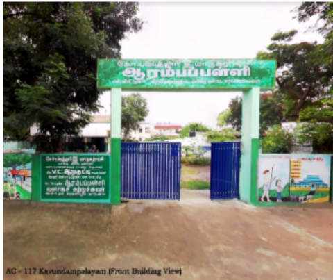
AG - 117 Kavundampalayam (Front Building View)
