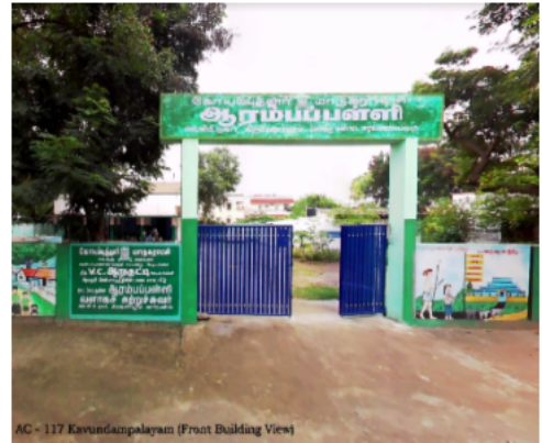
AG - 117 Kavundampalayam (Front Building View)
