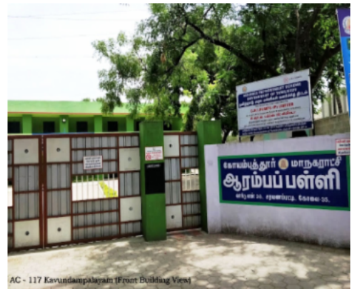
AC - 117 Kavundampalayam (Front Building View)
