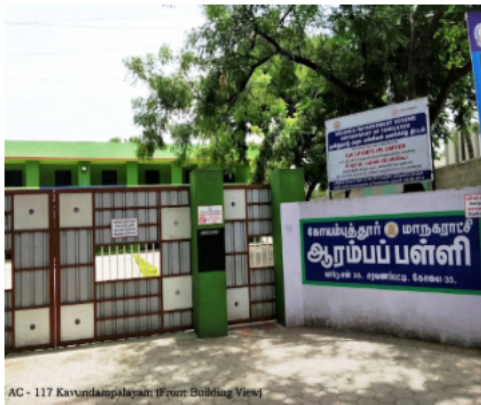
AC - 117 Kavundampalayam (Front Building View)
