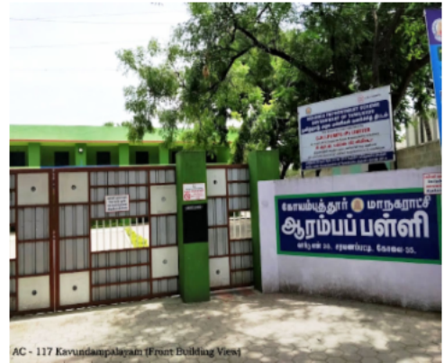
AC - 117 Kavundampalayam (Front Building View)
