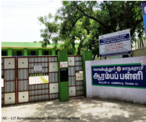
AC - 117 Kavundampalayam (Front Building View)
