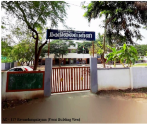
SC - 117, Kuvendampalayam (Front Building View)
