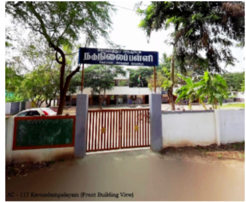
SC - 117, Kuvendampalayam (Front Building View)
