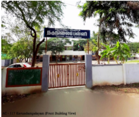
SC - 117, Kuvendampalayam (Front Building View)
