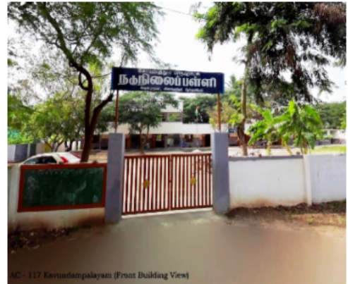
SC - 117, Kuvendampalayam (Front Building View)
