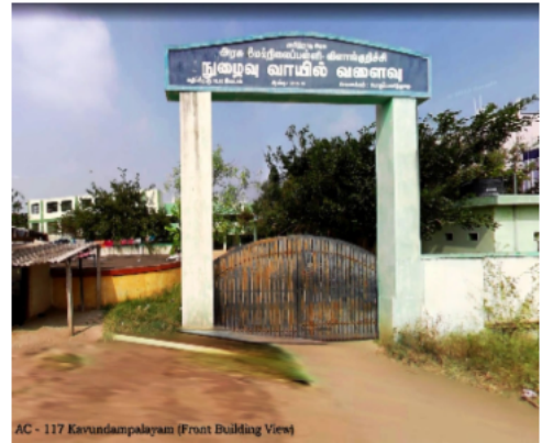
AC - 117 Kavundampalayam (Front Building View)
