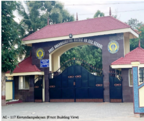
AC - 117 Kavundampalayam (Front Building View)
