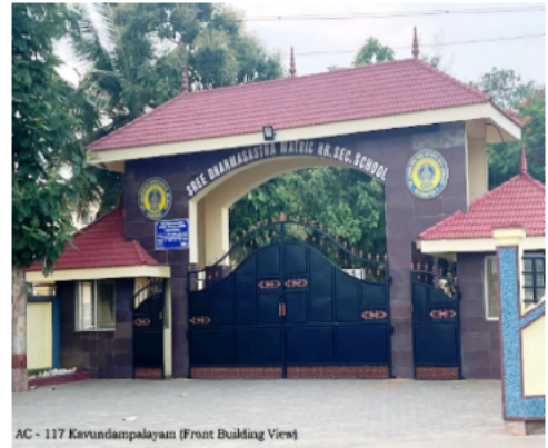
AC - 117 Kavundampalayam (Front Building View)
