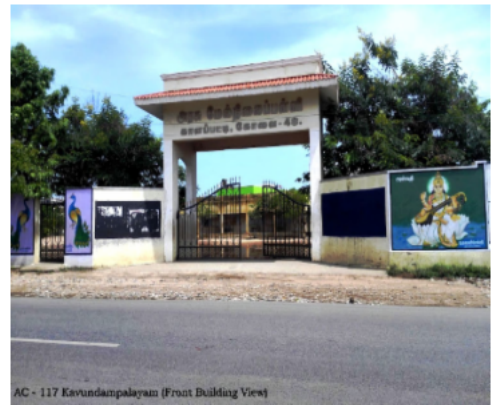
AC - 117 Kavundampalayam (Front Building View)
