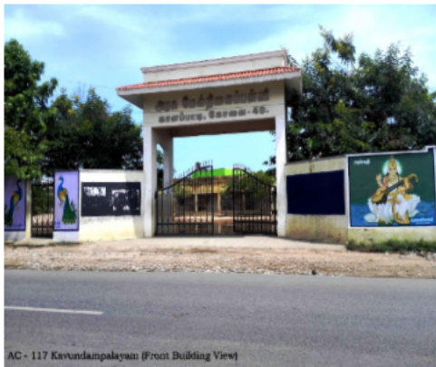
AC - 117 Kavundampalayam (Front Building View)
