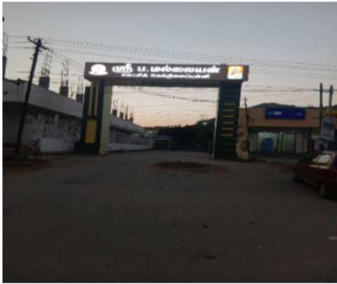
Polling Station Building Front View
