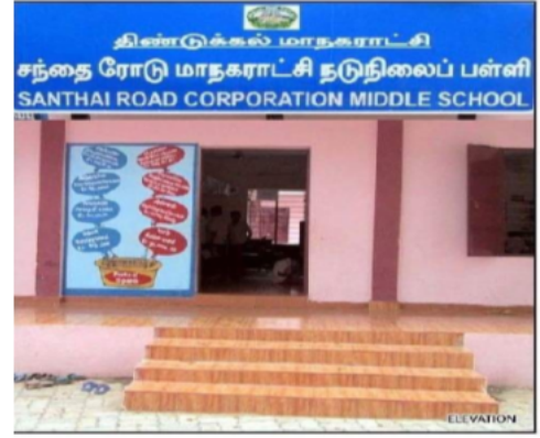
Polling Station Front View
