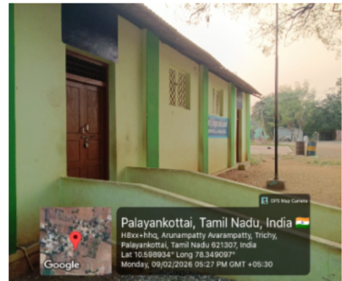
Polling Station Front View
