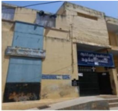
FRONT VIEW / MAIN ENTRY
