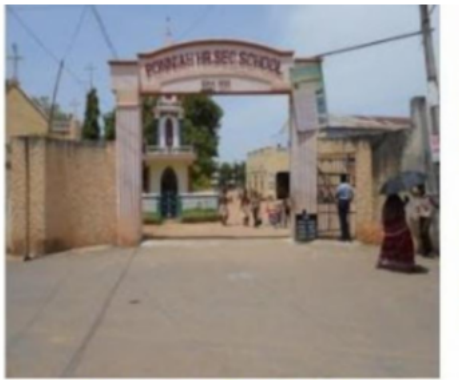
FRONT VIEW –( MAIN ENTRY)
