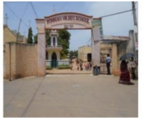
FRONT VIEW –( MAIN ENTRY)
