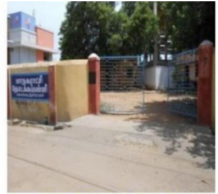
FRONT VIEW -( MAIN ENTRY)
