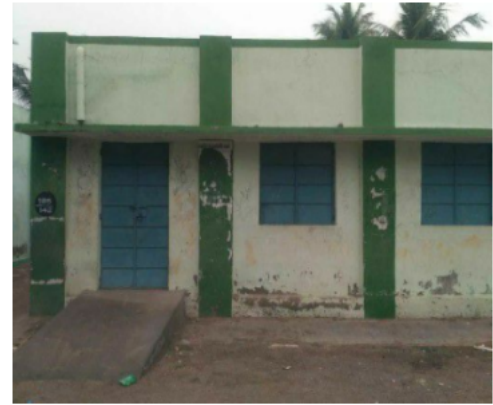
Polling Station Front View
