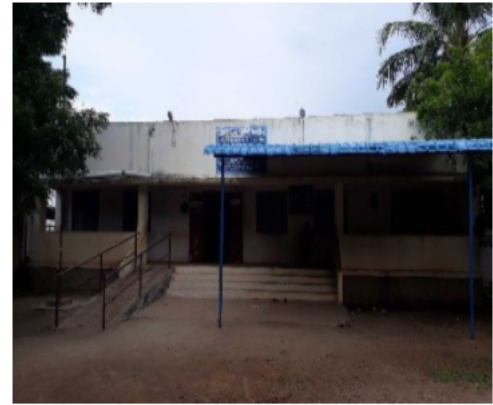
Polling Station Front View
