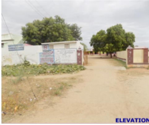
Polling Station Building Front View
