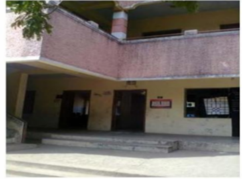
Elevation of Polling Station
