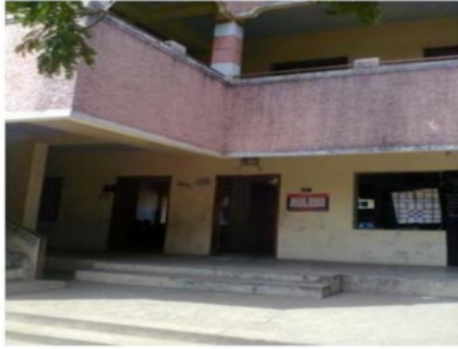
Elevation of Polling Station
