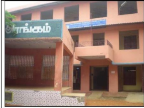
Elevation of Polling Station
