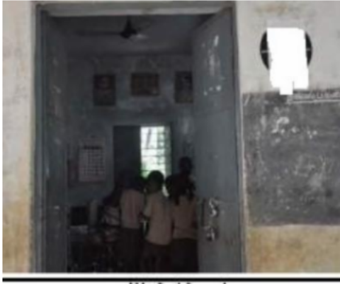
Polling Station Building Front View
