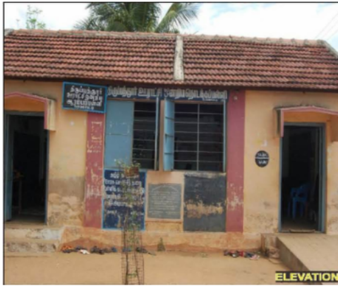
Polling Station Building Front View
