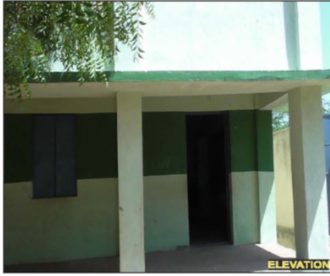
Polling Station Building Front View
