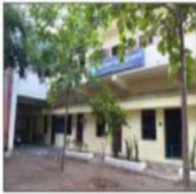
Polling Station Building Front View
