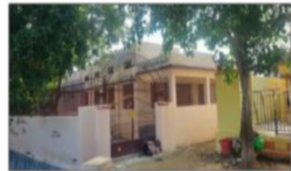
Polling Station Building Front View
