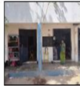
Polling Station Front View
