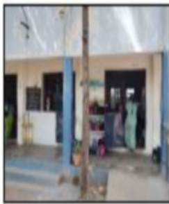
Polling Station Building Front View
