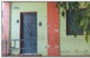
Polling Station Building Front View
