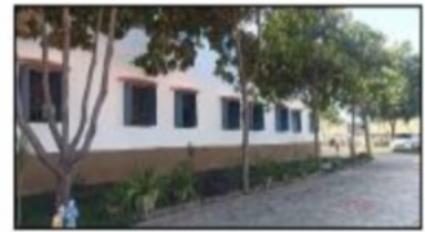
Polling Station Front View
