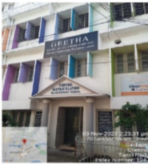
Polling Station Building Front View
