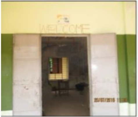
Polling Station Building Front View
