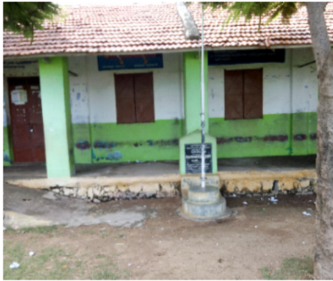
Polling Station Building Front View
