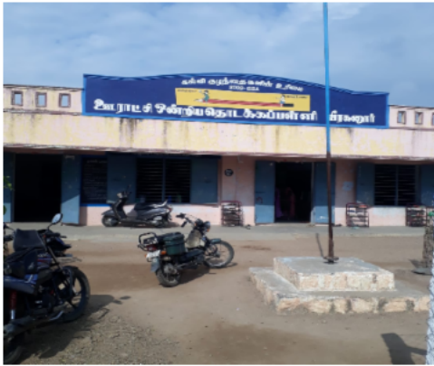
Polling Station Building Front View
