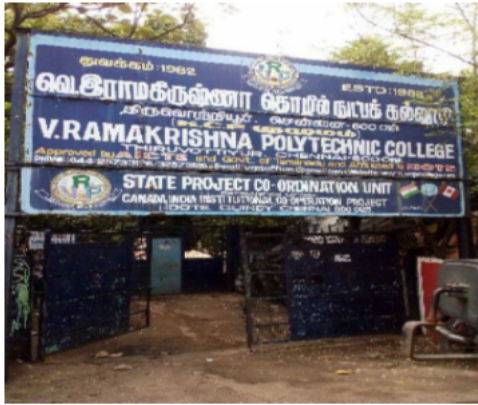
Polling Station Building Front View
