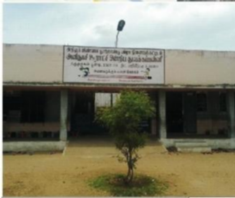
Polling Station Building Front View
