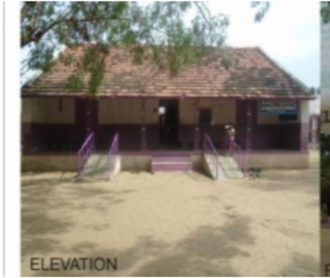
Polling Station Building Front View
