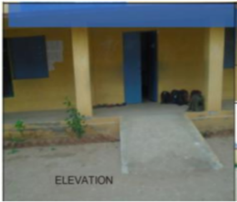
Polling Station Building Front View
