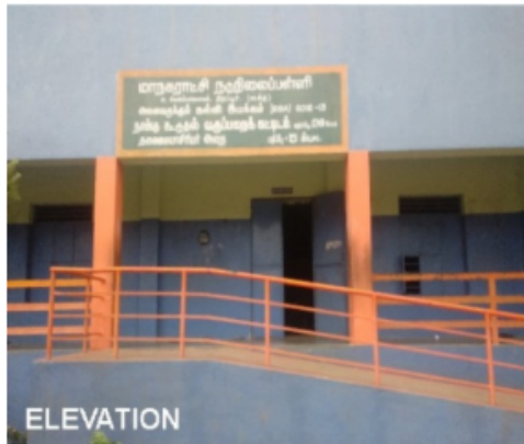
Polling Station Building Front View
